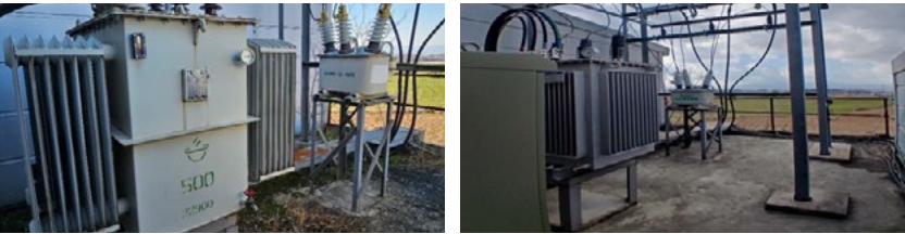
Before and After Transformer Replacement
