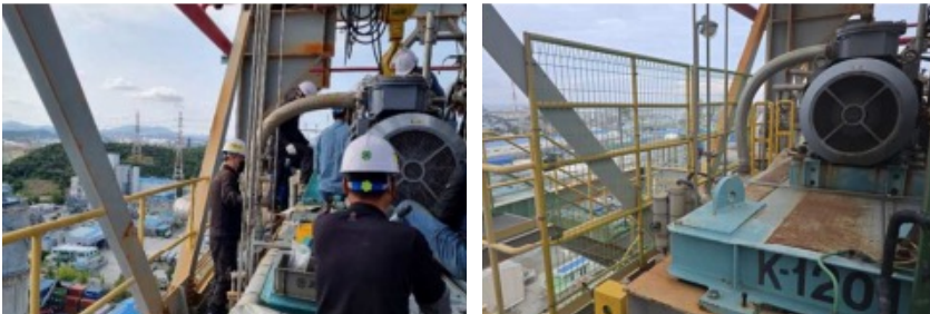
Fall Protection: Before and after safety fence reinforcement improvements
