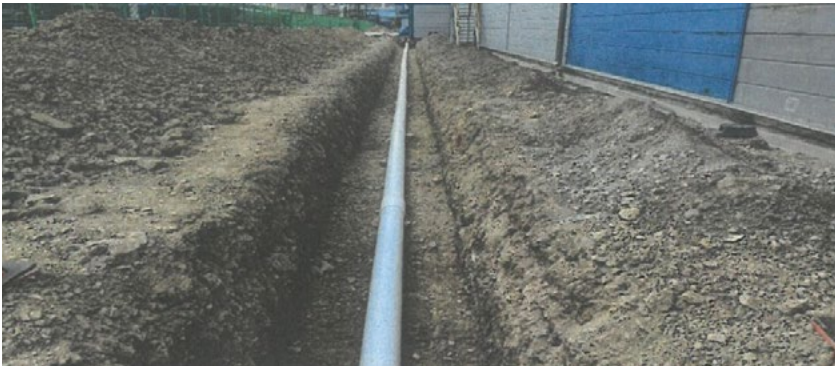
Typhoon and Flood Prevention: Before and after Additional Stormwater Drainage Installation
